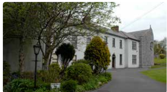
Forster Street building will be renovated to house the new Domestic Abuse Service.
